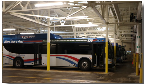
All BARTA vehicles can fit inside expanded facility helping with cleanliness of the vehicles.
