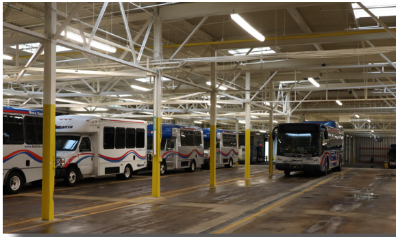
Inside renovated facility with improved lighting.
