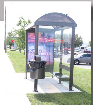
Solar Panel Bus Shelter on 5th Street Highway near Bellevue Avenue intersection.
